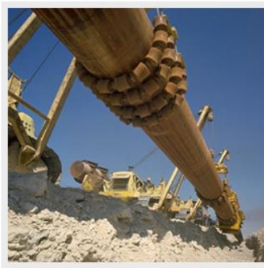
Buried metal structures
